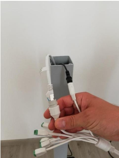
6. Insert the cables inside the body of the post and secure with the remaining screws of the cover.
